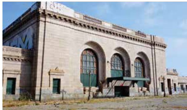
Old 16th Street Station, Oakland, 2013. 71 The abandoned 16th Street Station is slated for redevelopment as part of the Wood Street Development project. Photograph courtesy of Richard Johnstone, Flickr Creative Commons, under the license: http://creativecommons.org/licenses/by-nc-nd/2.0/ .
